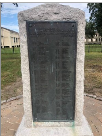
Monument with green patina and salt efflorescence of granite - Photo by Elizabeth Schexnyder
